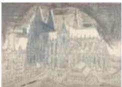
Renovation of the cathedral in Cologne
