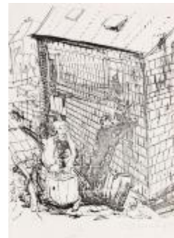
Building a house
